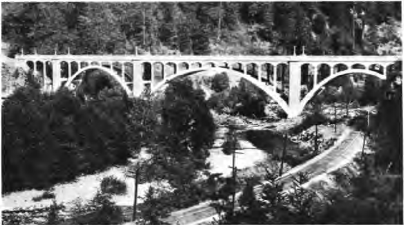
Bridge across Sacramento River at Dunsmuir.
